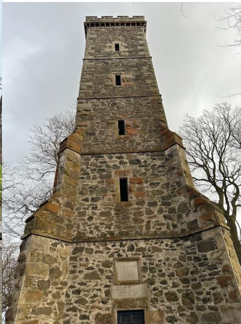
Corstorphine Hill Tower erected in 1871
